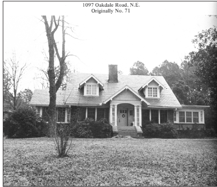
The house at 1097 Oakdale from the "Oakdale Road" book
