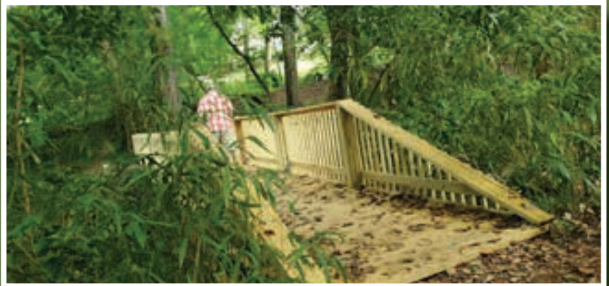
One of three new bridges across Lullwater Creek.
