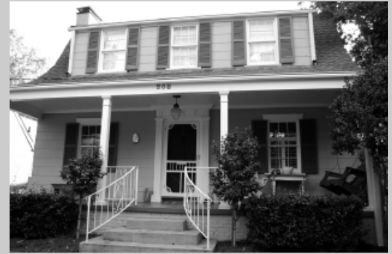
208 COVENTRY ROAD, DECATUR
