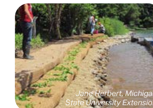
Bank stabilization and revegetation using soil lifts, shown on install day (left) and 2 years later (right).
